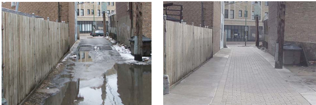
Typical Chicago Alley Vs. Retrofitted Green Alley
